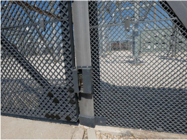
A long run of the 10-foot ENC FRP fence with the 45° anti-climb bill running continuously along the top. Open, hurricane-exposed Gulf Coast terrain made wind the governing load case.
