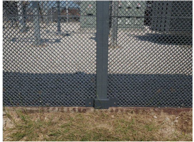
Post base plate concealed by an FRP cover where it meets the concrete apron.
