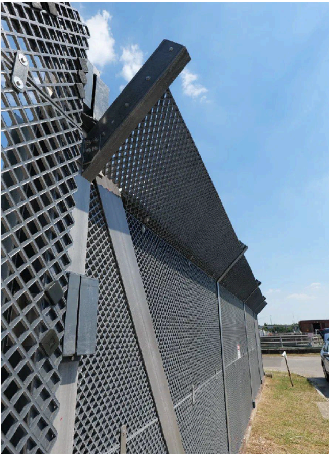
A long run of the 10-foot ENC FRP fence with the 45° anti-climb bill running continuously along the top. Open, hurricane-exposed Gulf Coast terrain made wind the governing load case.
