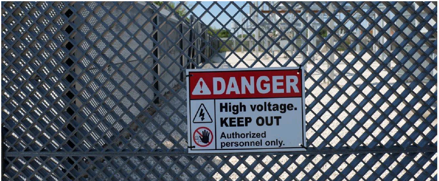
A long run of the 10-foot ENC FRP fence with the 45° anti-climb bill running continuously along the top. Open, hurricane-exposed Gulf Coast terrain made wind the governing load case.
