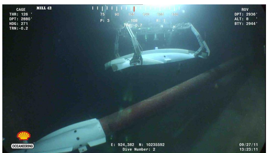
ROV equipped with ROV Strake Installation Tool installing strake
