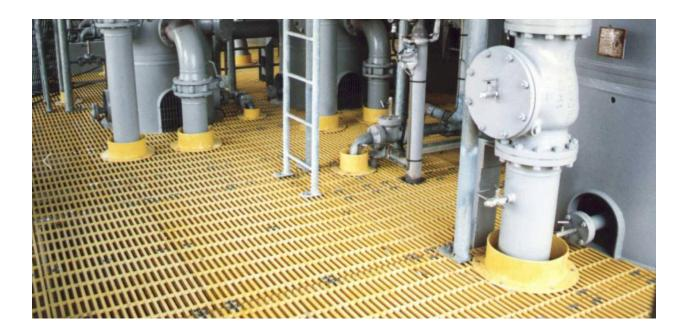
Here at AIMS Composites, we understand the importance of high-quality penetration collars when it comes to pipe integration. That's why we offer premium urethane penetration collars that provide superior durability and chemical resistance.
